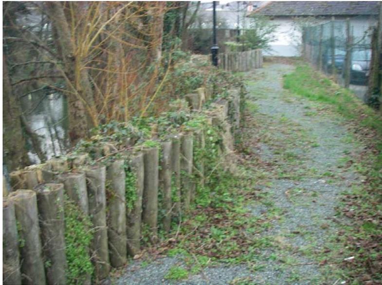
There is no clear maintenance regime in place to ensure the integrity of flood defence along the Western Cleddau in Haverfordwest. This position should be clarified and formalised as part of any proposed development in the flood plain.
