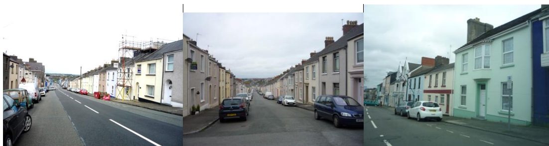
Properties at Church Street, Gwyther St, and Pembroke Street displaying varying degrees of unity but retain the original grid pattern (2017)
