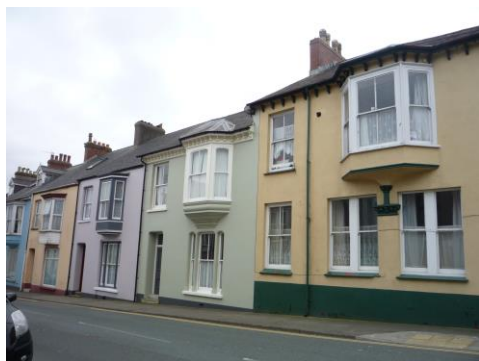
A variety of first floor oriel windows at Bush Street (2017)
