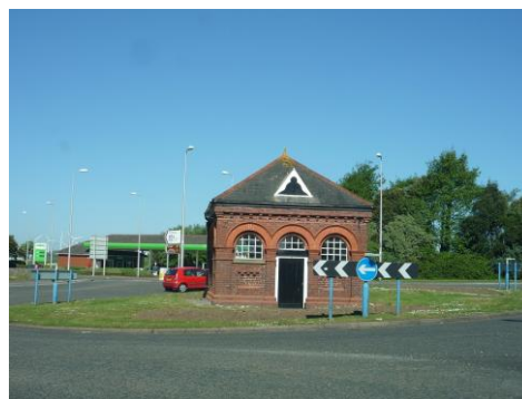
Former Pump House (2017)
