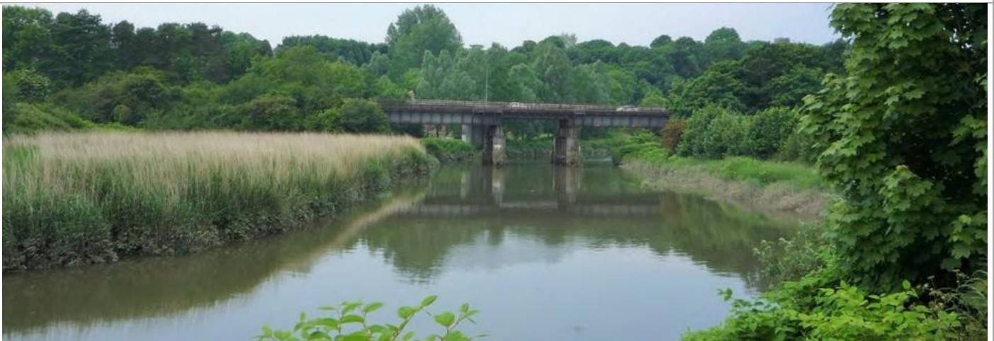
View along the Western Cleddau river to Haverfordwest at the railway and Freemans Way crossing.
